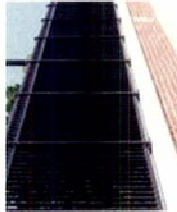
Tube steel fence along property edge
