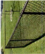
Chain link fence at exercise areas
